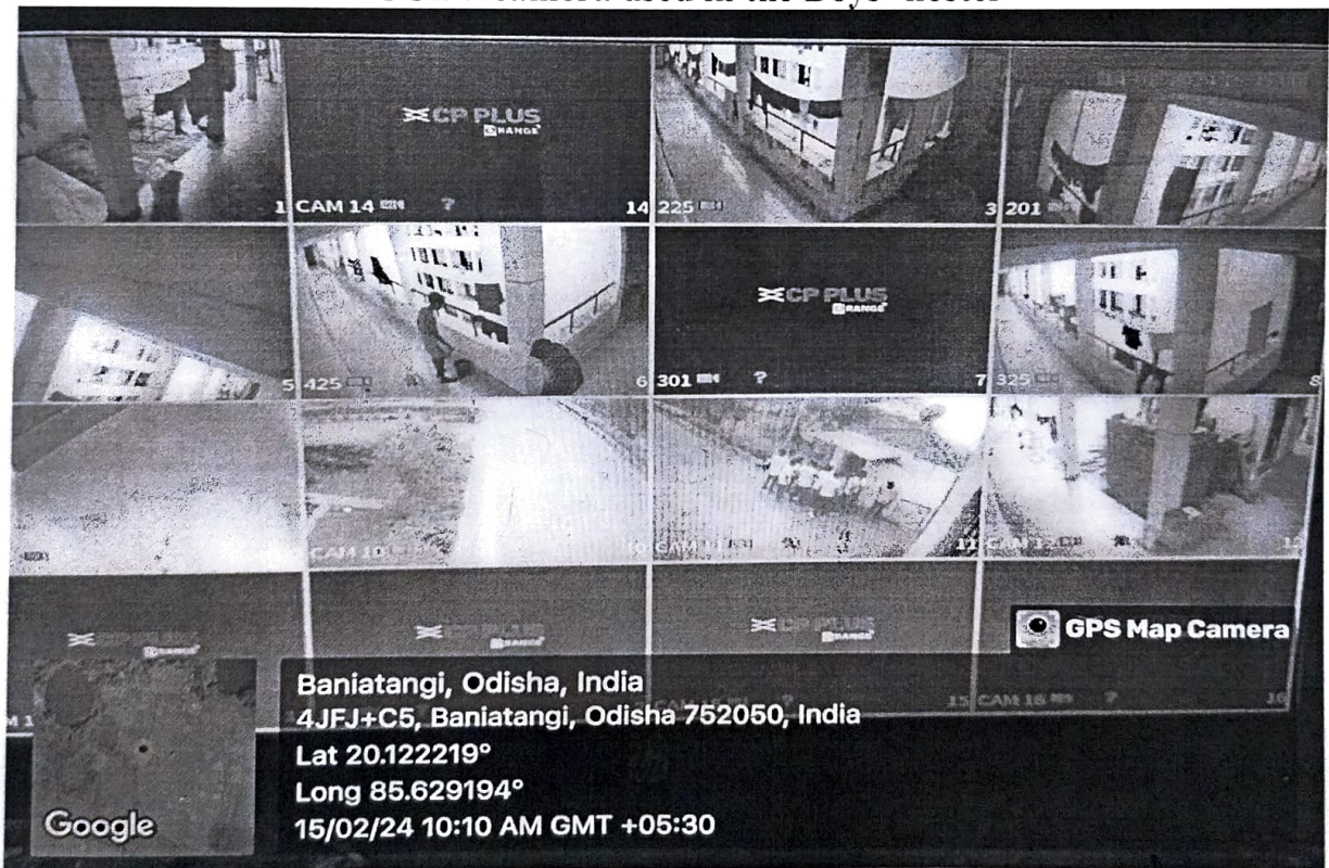
Display of the control room of CCTV cameras of Boys' hostel
